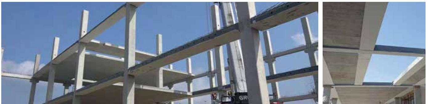
Industrial building, Wolomin, Poland
